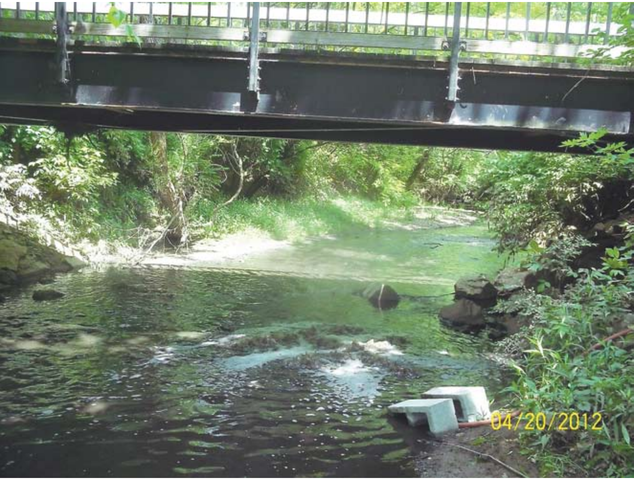
Air bubbles in Third Creek are created by the aeration system.
