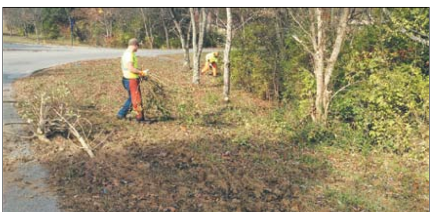
Workers trim brush from roads around the Mall exit.
