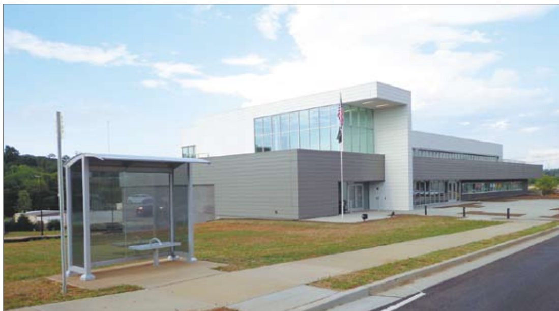
The new Public Works Building is on Morris Avenue near Middlebrook and houses most of the offices of that city department. There's a new bus stop there plus parking for the more than 265 employees.
