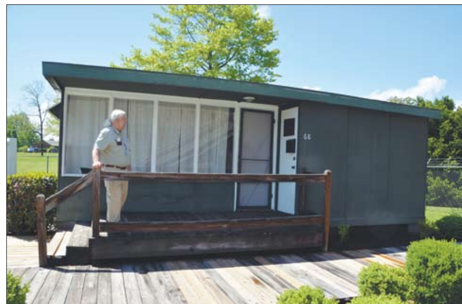
David Hackett, a volunteer at the American Museum of Science and Energy at Oak Ridge, stands in front of a B - 1 "alphabet house" on the grounds of the museum. This prefabricated two bedroom, 576 square foot house was one of many thousands factory built and trucked into the area to house workers at Oak Ridge.
