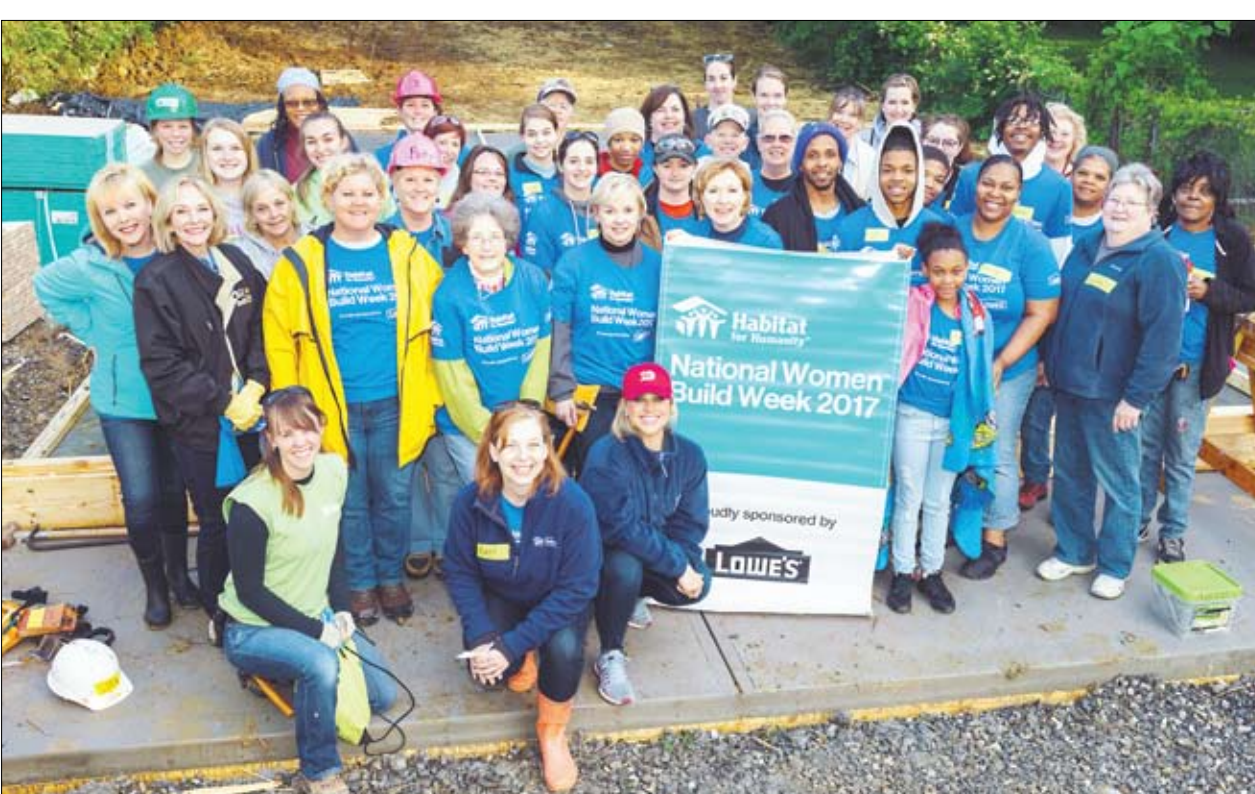
On Saturday, May 6, Knoxville Habitat for Humanity and Lowe's celebrated National Women Build Week by kicking off construction of a new home for future homeowner Kendra. Kendra is a Certified Nursing Assistant raising her three children in a tiny two-bedroom home that's in desperate need of repairs. Pictured with Kendra and her family are Women Build Honorary Chair Abby Ham, Knoxville Habitat Director of Development Angie Sledge, Director of Marketing & Communications April Timko and Women Build volunteers.
