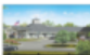
The new Morning Pointe Assisted Living building is set to open in the coming months. The building will provide assisted living services for the elderly in the community.
