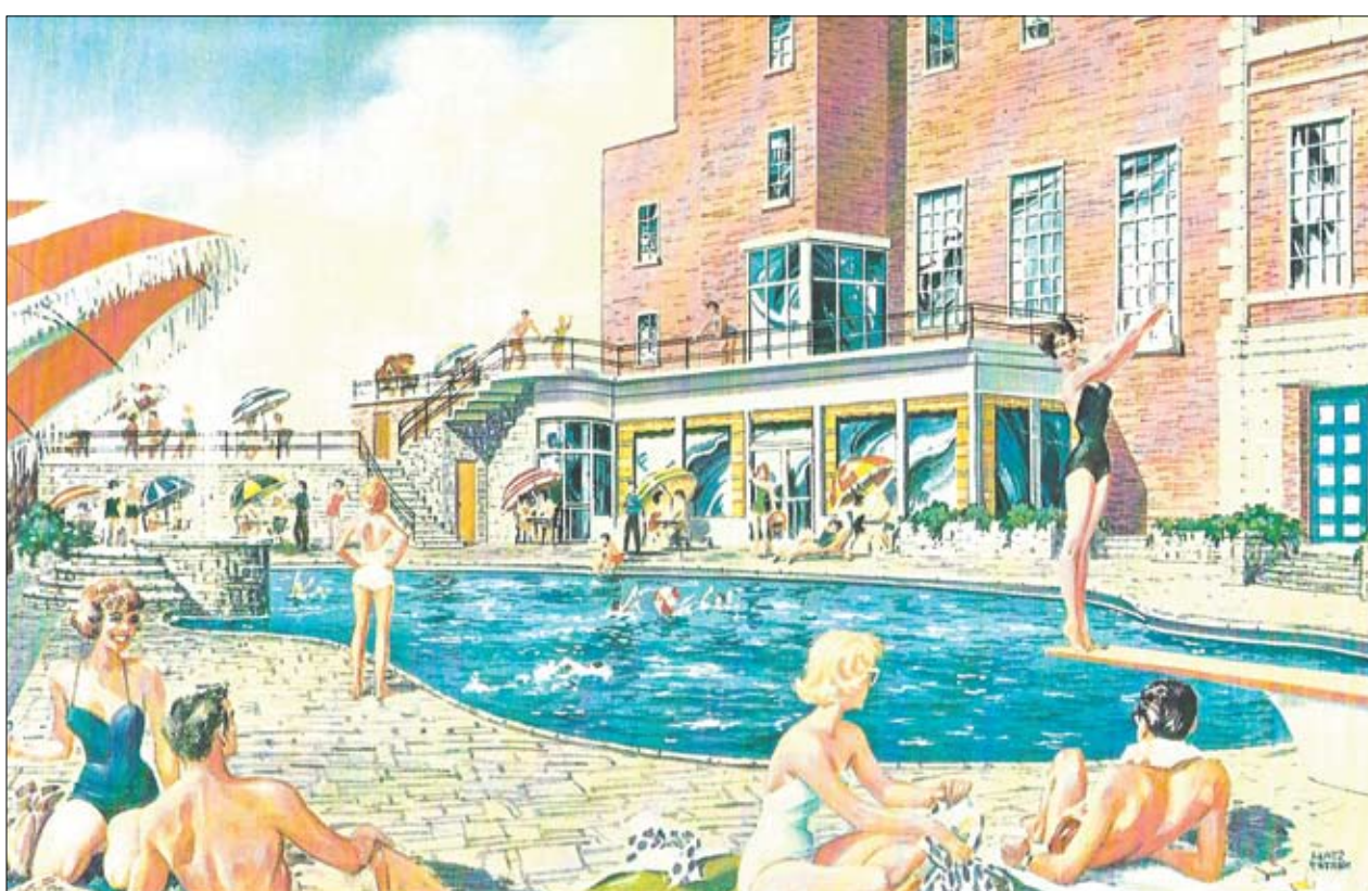
There's no sign of the pool that was advertised in the 1960s nowadays at the Andrew Johnson building. Like other features the building has been altered on the exterior and interior over the years. (Photo courtesy of the Knox County School Superintendent's office).
