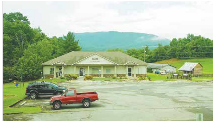
The Blaine City Halls sits along Indian Ridge Road just off Highway 11W. The community is growing and sits just south of Clinch Mountain between Knoxville and Rutledge.
