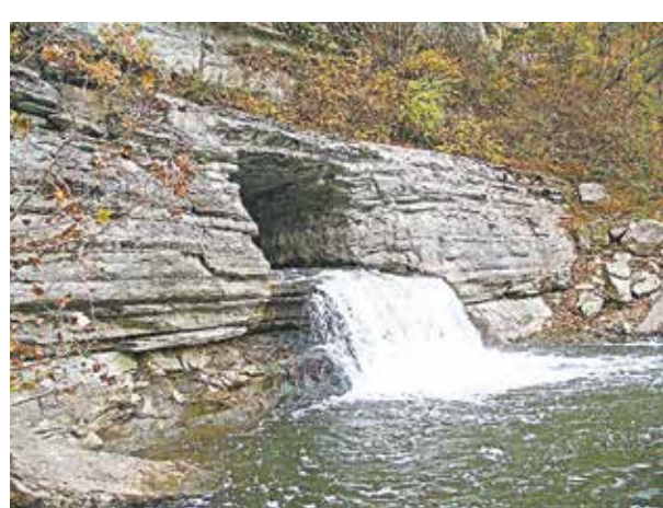
The Montgomery Bell Tunnel looks natural but was actually dug with dynamite and slave labor to redirect a portion of the Harpeth River. It's near Kingston Springs in West Tennessee.
