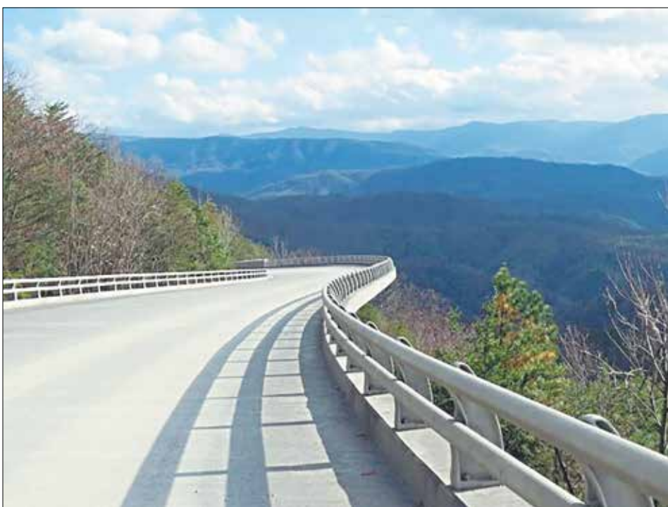
There are nine bridges along the "missing link" of the Foothills Parkway extension between Walland and Weirs Valley, some seeming to float on air. Photo from National Park Service.
