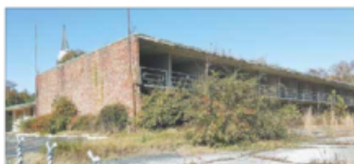
Abandoned for years and a neighborhood eyesore, the former motel property along Asheville Highway will come down and be replaced with affordable apartments if plans pass a second reading next week at the Knoxville City Council meeting.
