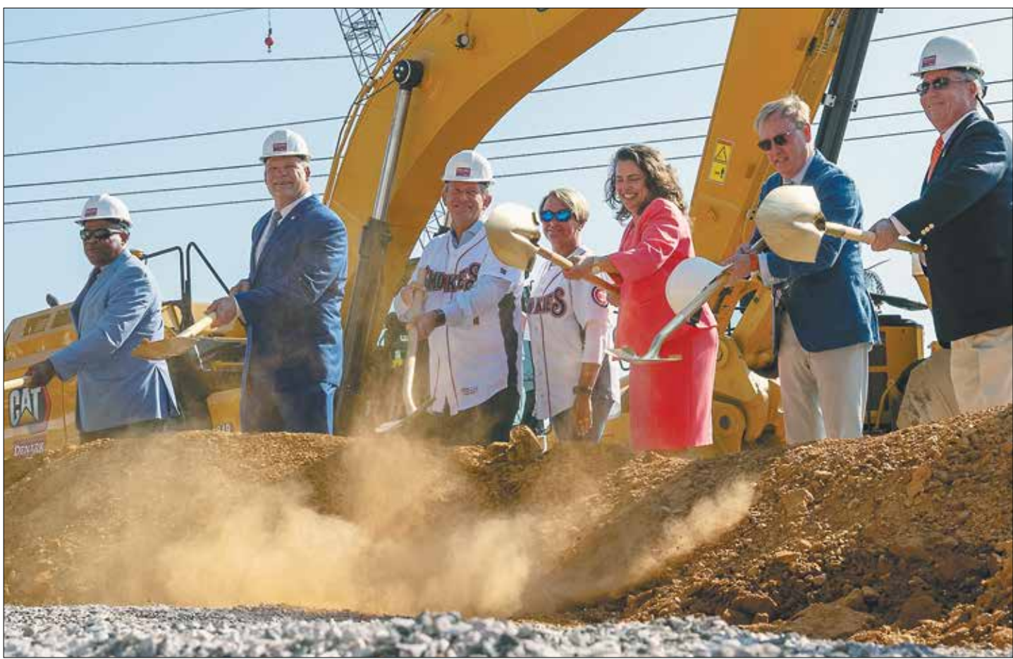
Randy and Jenny Boyd of Boyd Sports, center, flanked by Knox County Mayor Glenn Jacobs and Knoxville Mayor Indya Kincannon, officially break ground with elected officials and project partners on a multi-purpose stadium to be built in East Knoxville on the edge of the Old City. The stadium is scheduled to open in 2025. Photos provided by Moxley Carmichael.
