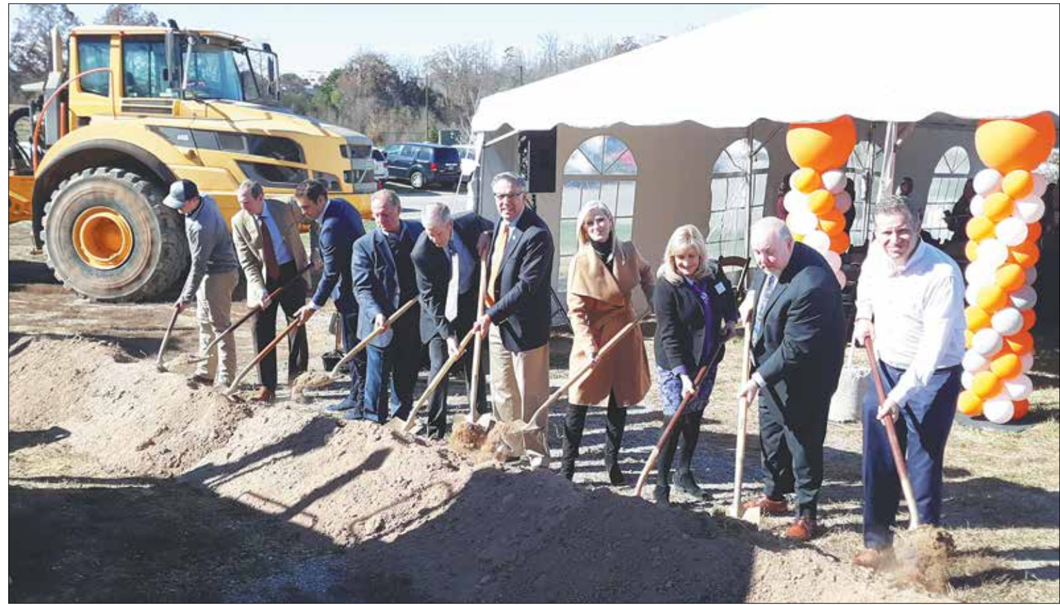
Taking part in the groundbreaking of Phase II of the Morning Pointe campus in Hardin Valley, were representatives from government, the private sector and advocates for memory loss care. Those included a members of the contracting team, ETSB LLC, of Harrison, Tenn.; CEO of Morning Pointe Senior Living Franklin Farrow (second from left); Riley Lovinggood of Senator Bill Hagerty's office (third from left); Mark Field, senior vice president of investor development with the Knox County Chamber of Commerce; Greg A. Vital, president of Morning Pointe Senior Living; Knox County Commissioner Kim Frazier; Janice Wade-Whitehead, president and CEO of Alzheimer's Tennessee; Rodney Holloman, pastor of Hardin Valley Church; and Kevin Parton, Knox County Health Department Senior Director (far right).
