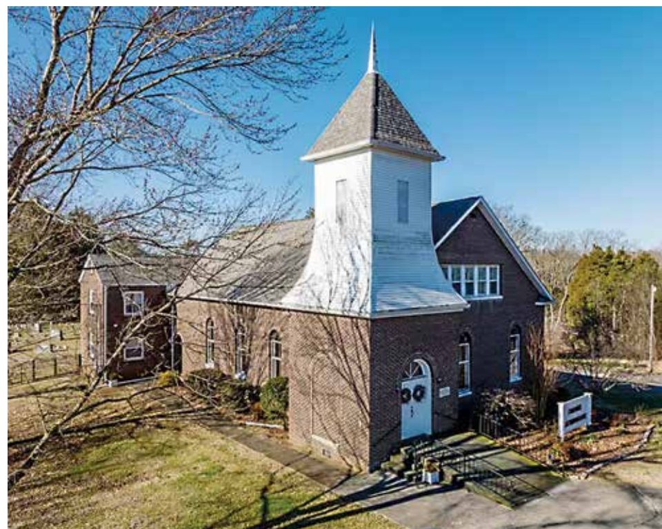
The Friendsville Church reflects the Quaker settlements in our area and the word "friends" appears in names here and there across the nation.
