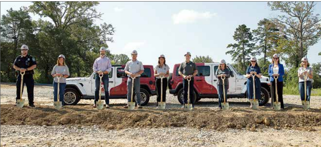
Construction is underway at the new KTVAECU location at 7605 Strawberry Plains Pike in Knoxville. The branch will be completed in early 2027.
